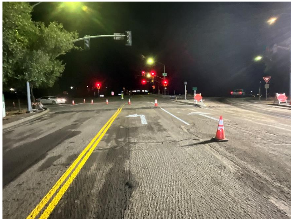
Pavement grinding
