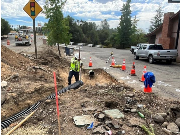
Adding new drainage system.
