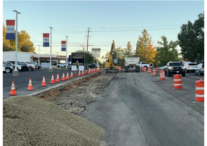
Pavement grinding
